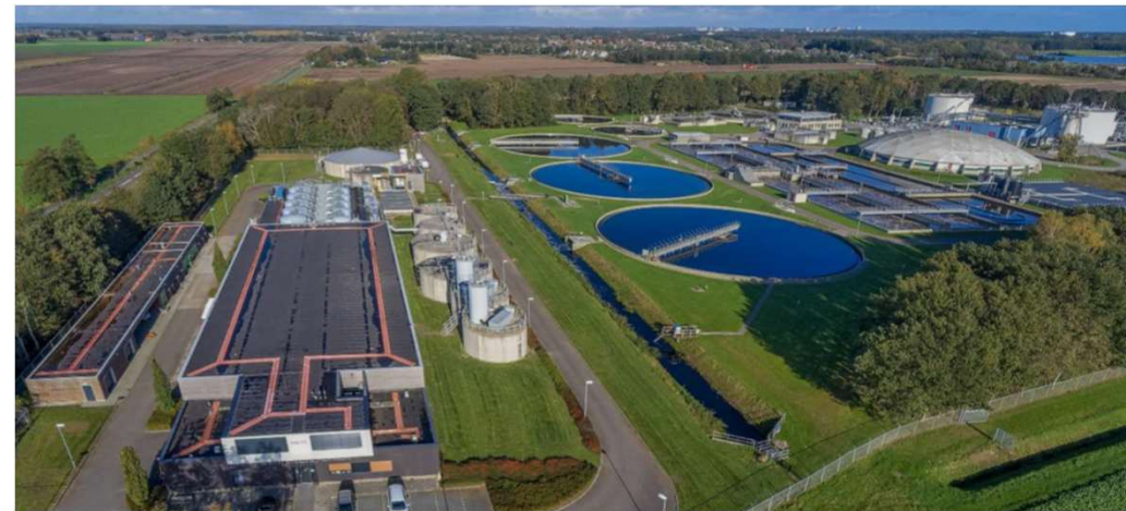
Located at WWTP Emmen – UPW
