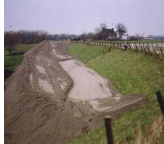
Temporary reinforcement
