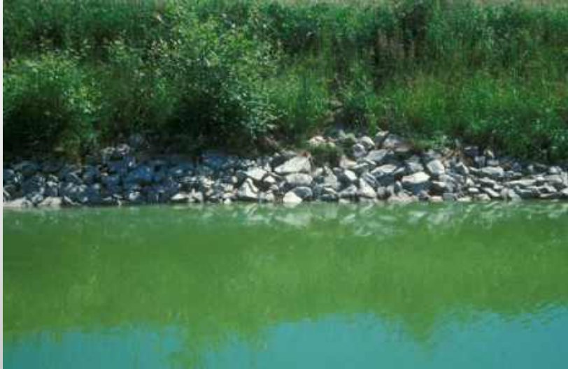
Protection of the shores with a layer of heavy stones
