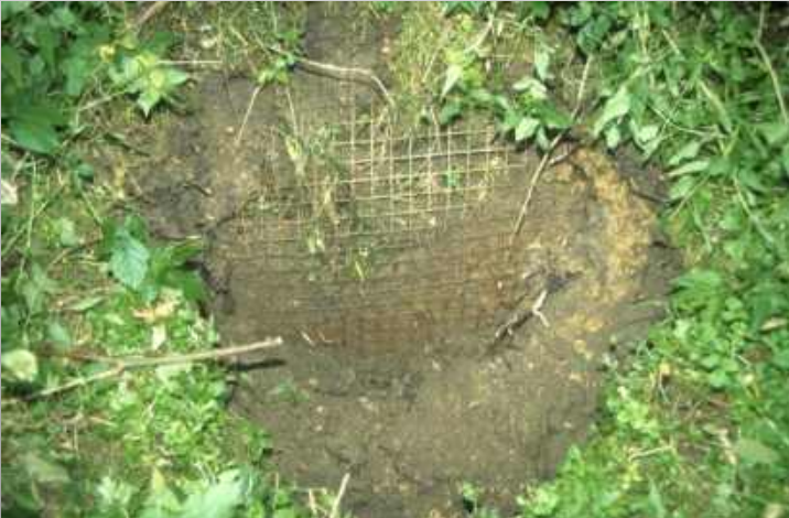
Wire mesh dug in the banks
