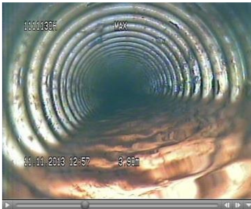
Figure 5. Good dewatering by drain, installed in Texel sea clay (photo: L C P M Stuyt, 11 November 2013)
