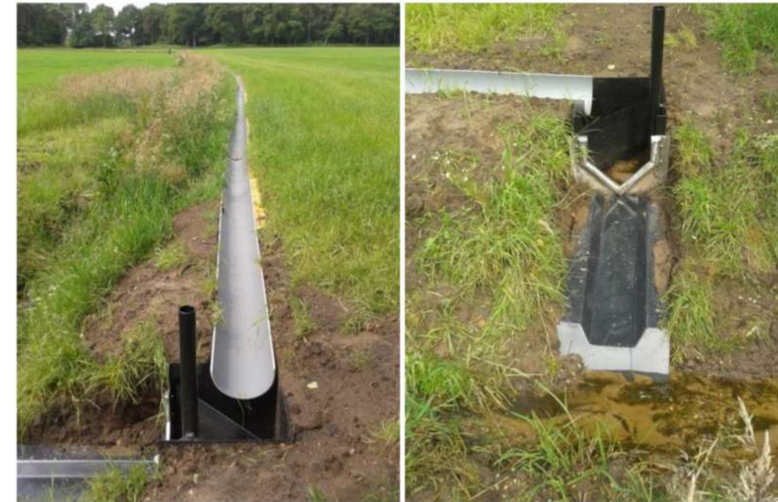
Figure 2: Surface runoff collecting gully.
