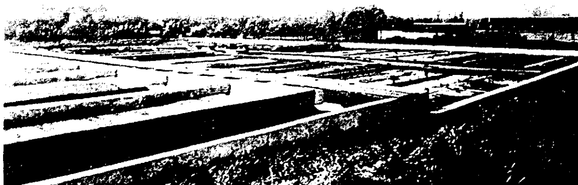
Figure 1 Voorburg sewage treatment plant; trickling filters (1906).
