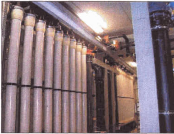
Figure 5 - Tube membrane installation (X-Flow)
