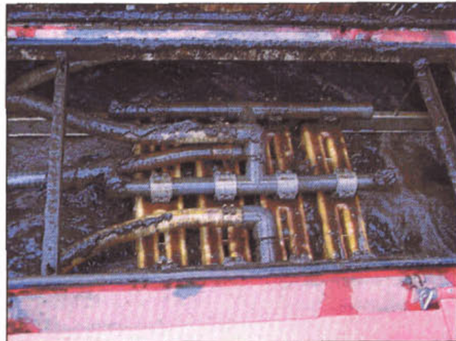
Figure 30 - Top view Zenon membranes
