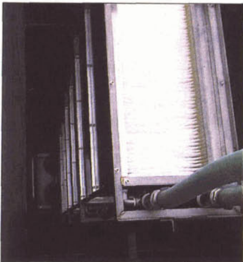
Figure 26 - Top view Mitsubishi element
