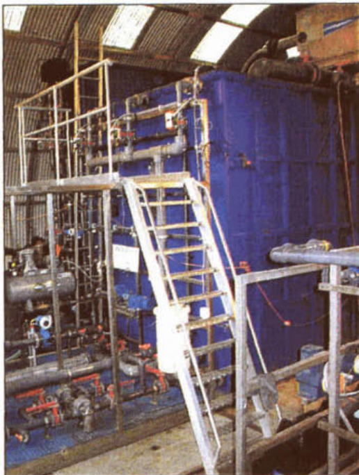
Figure 24 - Kubota DD system in Beverwijk
