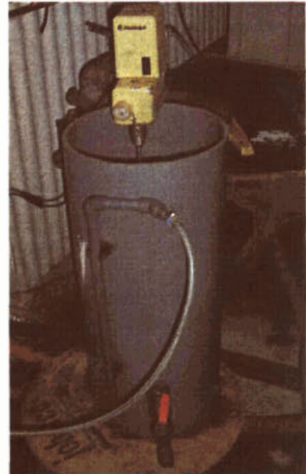
Figure 2 - Diffused air aeration setup
