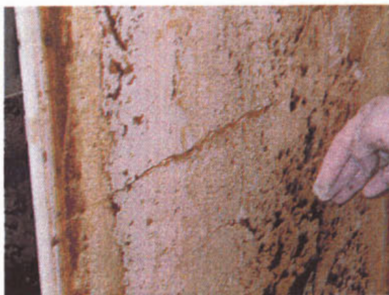
Figure 2 - Extreme Calcium Carbonate (chalk) scaling in an industrial MBR
