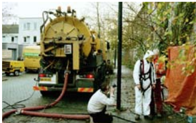
ONTMANTELING VAN DE COMPOSTERINGSTOILETTEN IN NOVEMBER 2000 (WEBSITE GROENE DAK)
