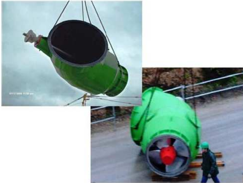
Figure 3: Installation of Kaplan turbine in Seine Aval WWTP (Nitrification Unit)
