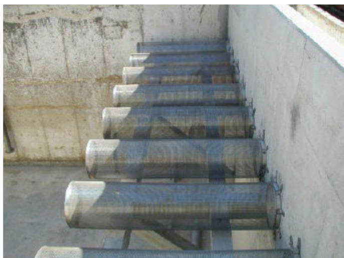
WEDGE-WIRE SCREENS AFTER INSTALLATION
