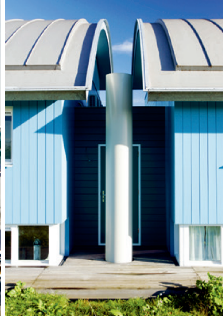
The mooring posts in which the houses can move up and down according to the water level (photo: Dura Vermeer)
