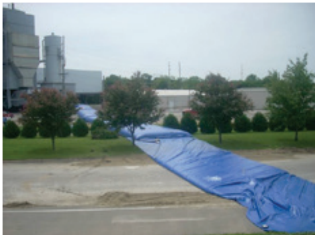
Moveable dams, filled with water or sand (image: atelier GROENBLAUW)
