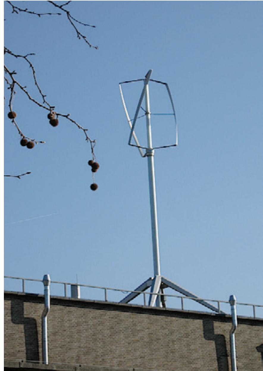
Vertical-axis wind turbine Turby (photo: VanBuren)
