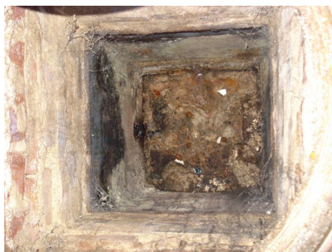
Figuur 9.13 Vetafzettingen in put 54r0152 (links) en put 54r0149 (rechts)
