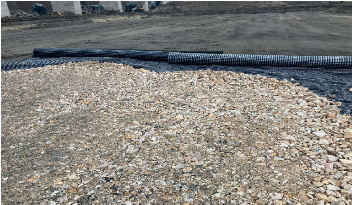
PHOTO 5-3 STRUCTURE OF A MIXED AGGREGATE PLATFORM FOUNDATION REINFORCED WITH A GEOSYNTHETIC (HORIZONTALLY-LAID GEOGRIDS)
