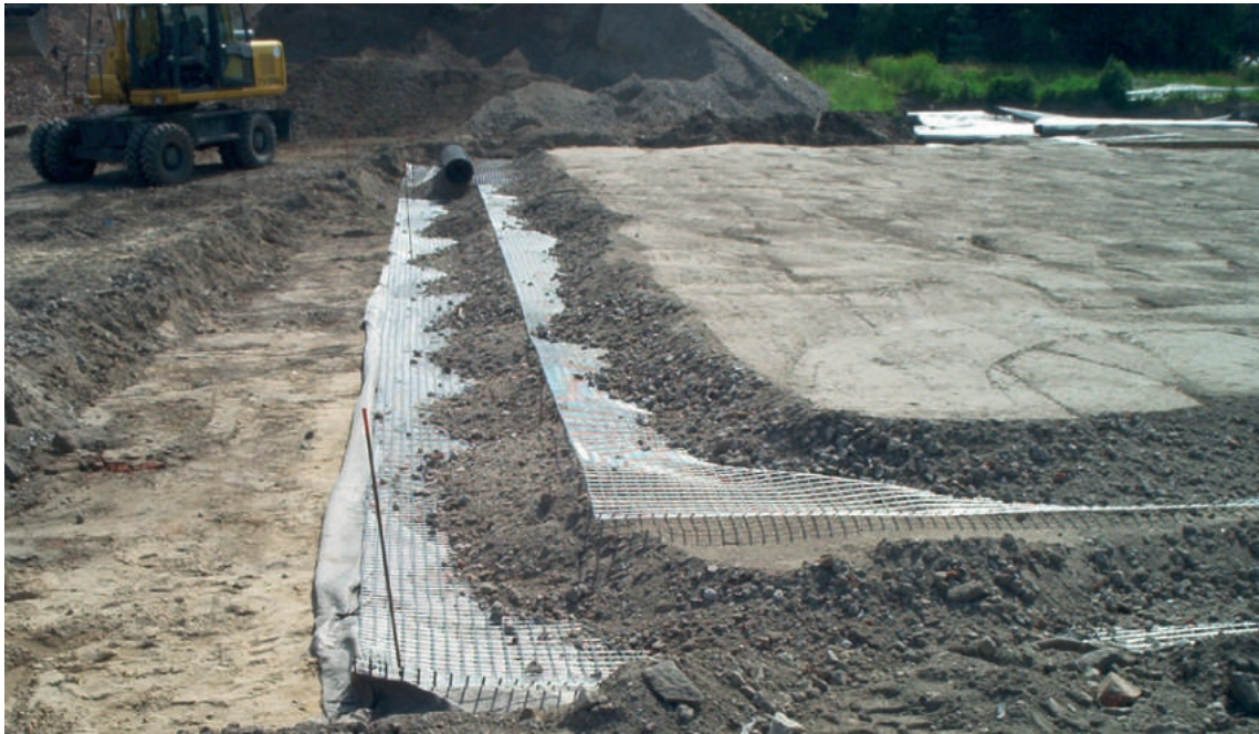
PHOTO 5-2 STRUCTURE OF A HARDSTAND FOUNDATION USING A MIXED AGGREGATE REINFORCED WITH A GEOSYNTHETIC (MULTIPLE LAYERS OF HORIZONTALLY-LAID GEOGRIDS)
