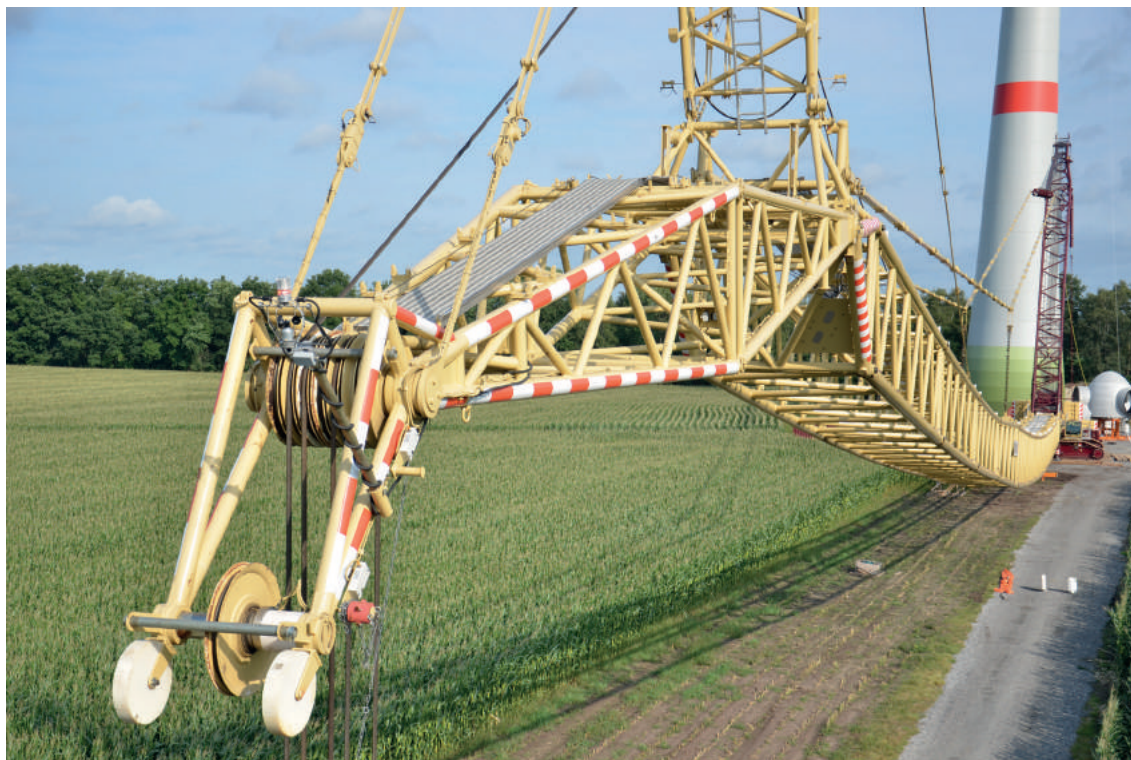
PHOTO 3-11 ERECTING THE BOOM OF A DEMAG CC 3800-1
