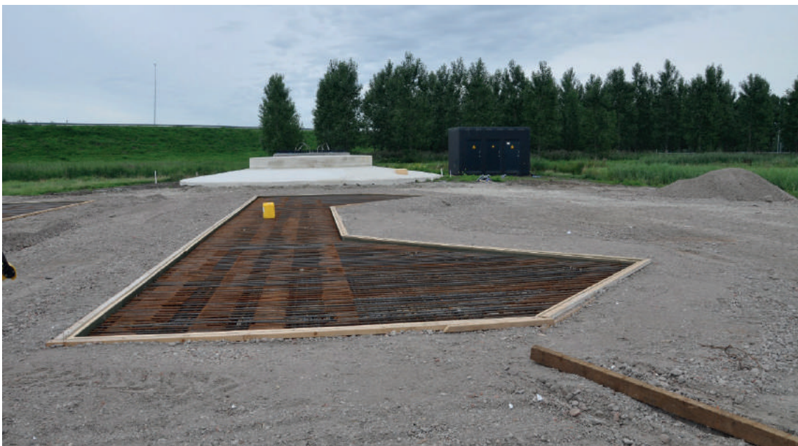
CONCRETE-FOOTED PILE FOUNDATION, STEEL REINFORCEMENT IN PROGRESS
