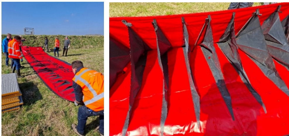
Figure 2.75 The connection of two modules requires the individual layers to be joined using hook-and-loop fasteners. This process is labour-intensive and susceptible to assembly errors, as one or more layers can easily be overlooked during installation.
