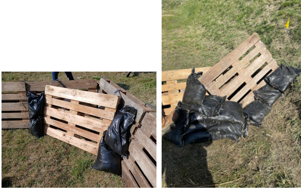
Figure 2.18 Sandbags are used to fill gaps at corners and slope transitions.
