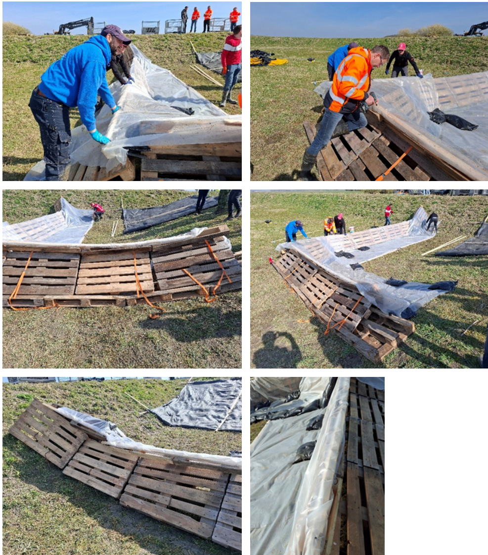
Figure 2.27 The timber battens are rolled into the plastic sheeting towards the dry side of the structure. This results in a smooth and wrinkle-free surface, allowing overtopping water to pass more readily over the barrier.
