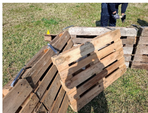
Figure 2.16 An L-shaped configuration of three-pallet modules. The corner is reinforced using an additional pallet fixed in place with metal clamps.
