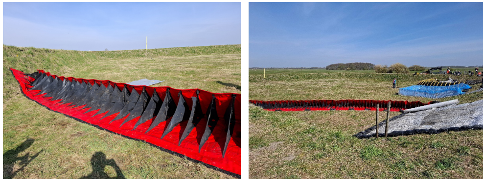
Figure 2.81 The BFW system is positioned diagonally within one corner of the basin, connecting the two embankment slopes.
