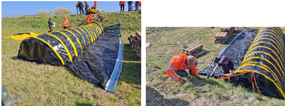
Figure 2.41 The TubeBarrier anchored against the slope by means of ratchet straps.
