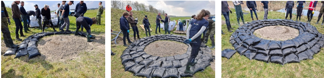
Figure 4.6 Construction of a sandbag ring dike, with each layer of sandbags compacted by walking on it to ensure good interlocking between the bags. The sandbags should not be tamped.
