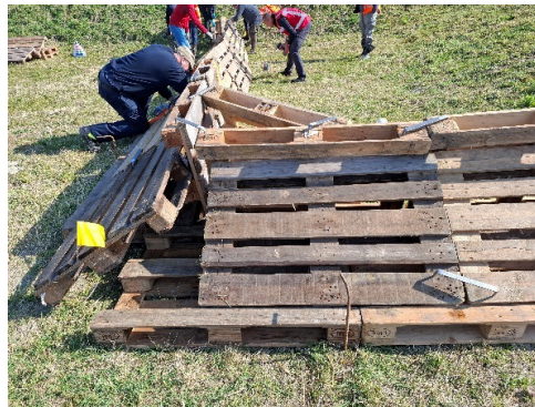
Figure 2.15 The three-pallet modules are interconnected in a staggered bond arrangement using metal clamps.
