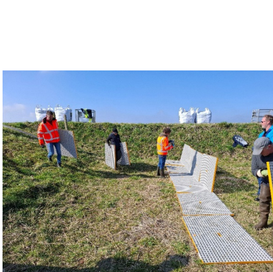
Figure 2.52 Installation of the Haawal system with a curved alignment.
