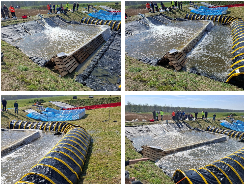
Figure 2.34 Performance test of the Euro pallet barrier during the second day of the exercise. The barrier remained stable under overtopping conditions, with no signs of instability or structural displacement.
