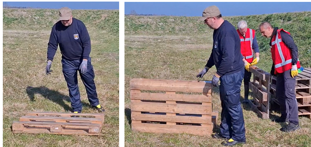
Inverted base pallet with an inclined pallet on the water-retaining side.
