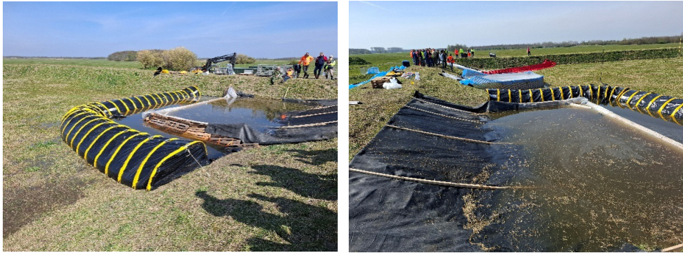
Figure 2.35 Following cessation of the water supply, the water level decreased only gradually, indicating a relatively high degree of watertightness of the barrier system.
