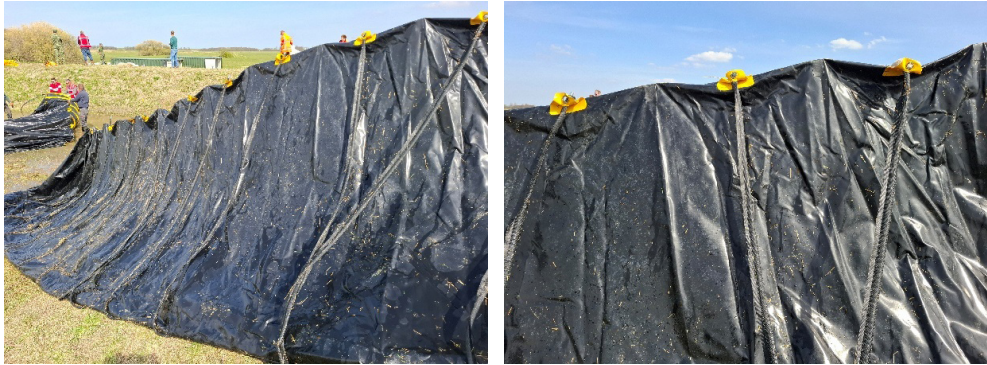
Figure 2.49 Folding, packing, and loading of the TubeBarrier.
