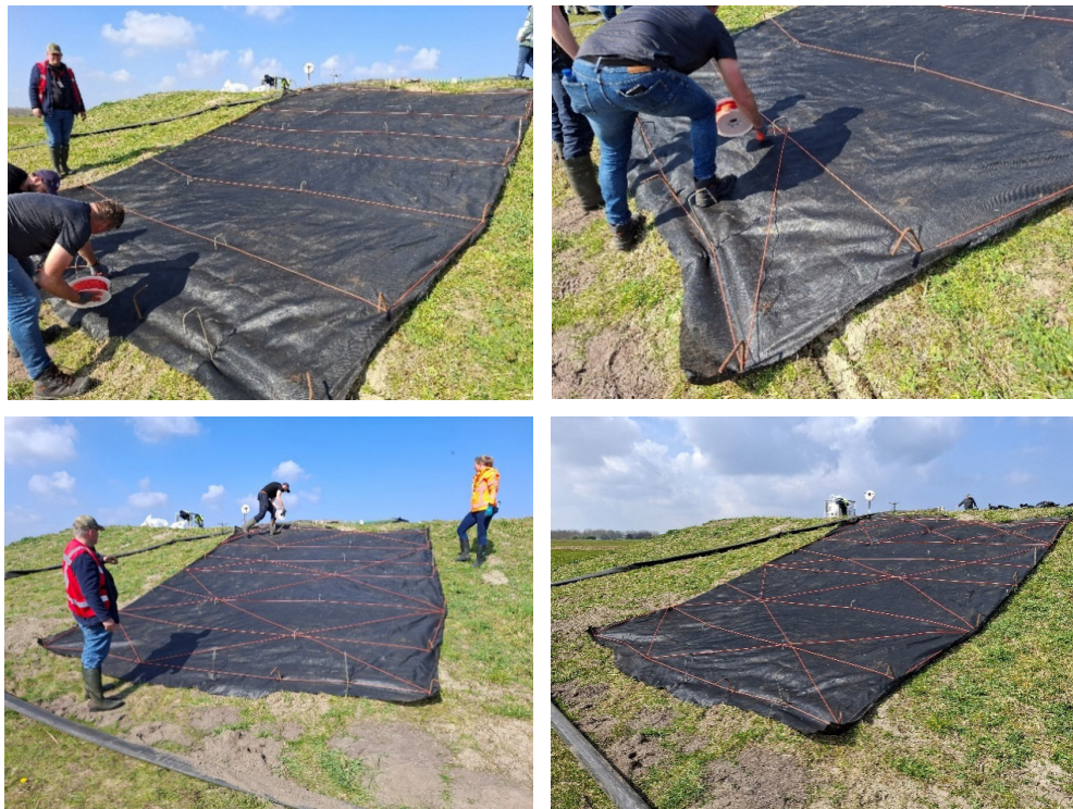
Figure 3.19 The geotextile is anchored by means of a high-strength rope that is looped around the anchoring pins. The rope is secured to an initial pin and subsequently unwound from the spool while being stretched across the geotextile surface.
