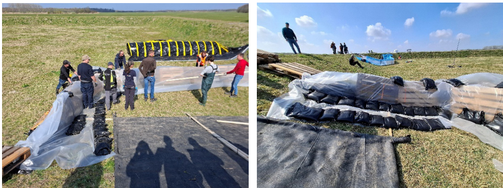
Figure 2.23 In the three-pallet configuration, the sheeting is primarily fixed in place using sandbags, both at the crest of the temporary flood barrier and directly against the pallets on the water-retaining side. The sheeting should be laid flat on the ground surface without wrinkles and ballasted along its perimeter with sandbags to prevent seepage beneath the barrier.
