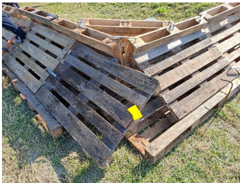
Figure 2.15 The three-pallet modules are interconnected in a staggered bond arrangement using metal clamps.
