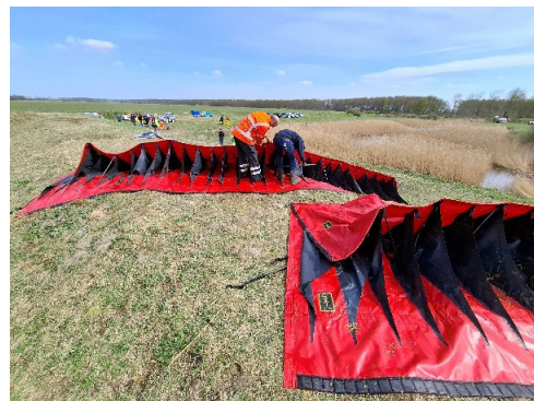
Figure 2.85 Although the grass had been cut approximately three weeks before the exercise, a considerable amount of vegetation became trapped in the BFW system during deployment. The subsequent cleaning of the system was found to be very labour-intensive.
