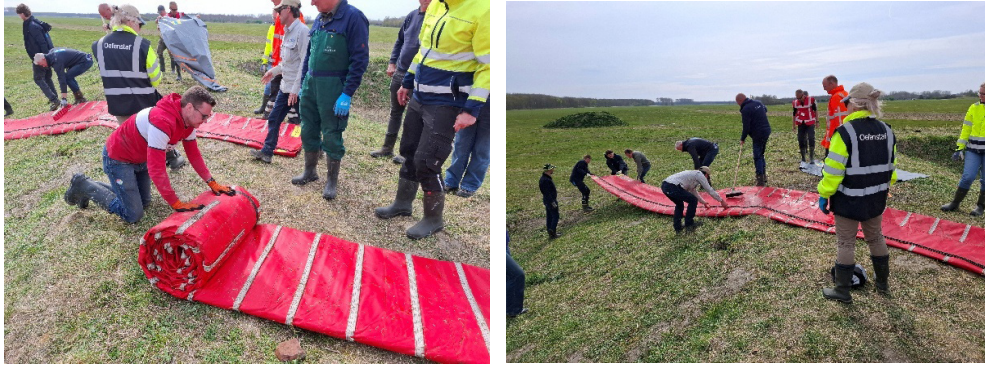
Figure 2.86 Rolling up and cleaning the BFW system.
