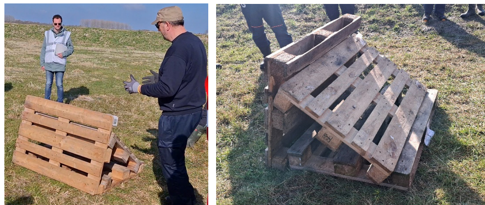
A third pallet is positioned behind the water-retaining pallet as a brace, with its base secured within the inverted pallet placed on the ground. The stability of the system against sliding is achieved through the frictional resistance of the inverted base pallet.
