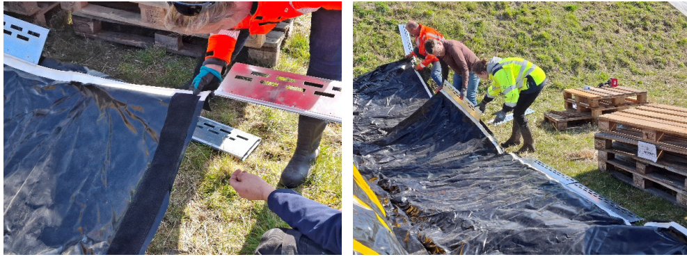
Figure 2.40 Installation of anchor plates in the water-side skirt of the TubeBarrier to mitigate underseepage.
