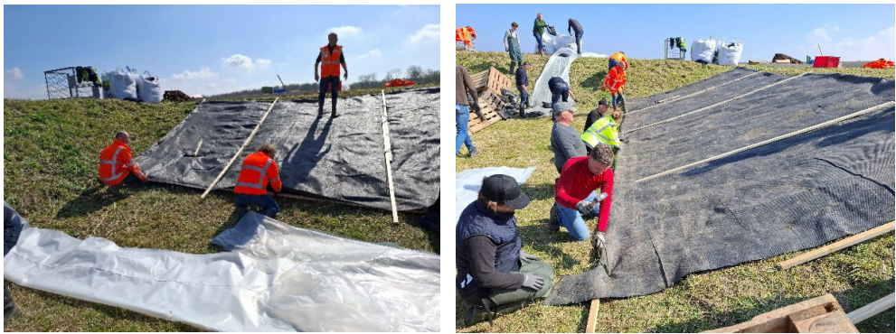
Figure 3.10 Timber battens are rolled into the four edges of the fabric and anchored into the ground using U-shaped staples.
