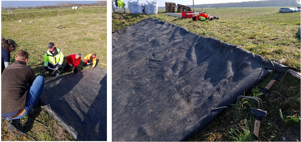
Figure 3.9 Geotextile Installation Using Timber Battens and U-Shaped Staples.
