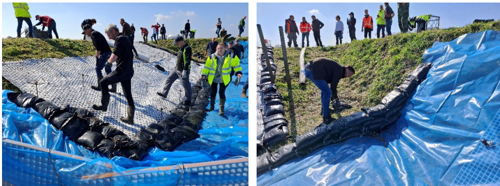
Figure 2.57 The outer edge of the membrane is ballasted with sandbags to reduce underseepage beneath the barrier. It is noticeable that the membrane still contains a considerable number of folds.
