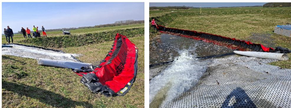
Figure 2.82 To improve the interface between the BFW and the dike slope, sandbags were positioned against the barrier. Additional sandbags were placed on the ground covering to provide ballast and enhance contact with the subsoil. Water was then introduced over the Tensar geogrid-reinforced section.
