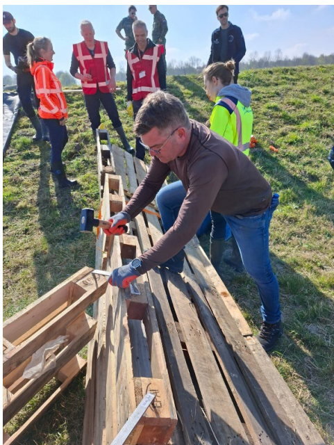
Figure 2.17 The Euro pallets are interconnected using robust, short steel U-clamps (staples).
