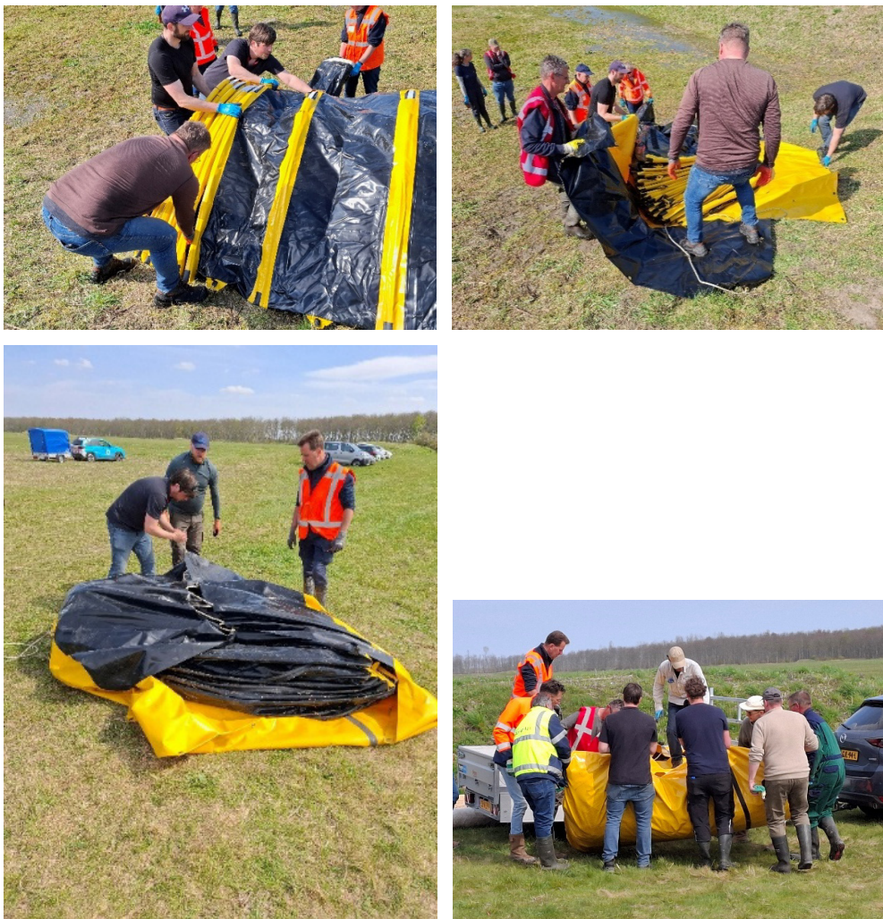
Figure 2.49 Folding, packing, and loading of the TubeBarrier.
