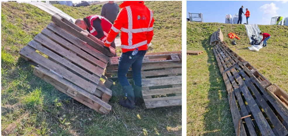
Figure 2.22 Placement of the Euro pallets at the slope transition is more challenging because the elements do not interlock properly in a staggered bond arrangement. Sandbags are required to seal the gaps to the ground surface and provide stability, while the pallets are secured together using steel staples.
