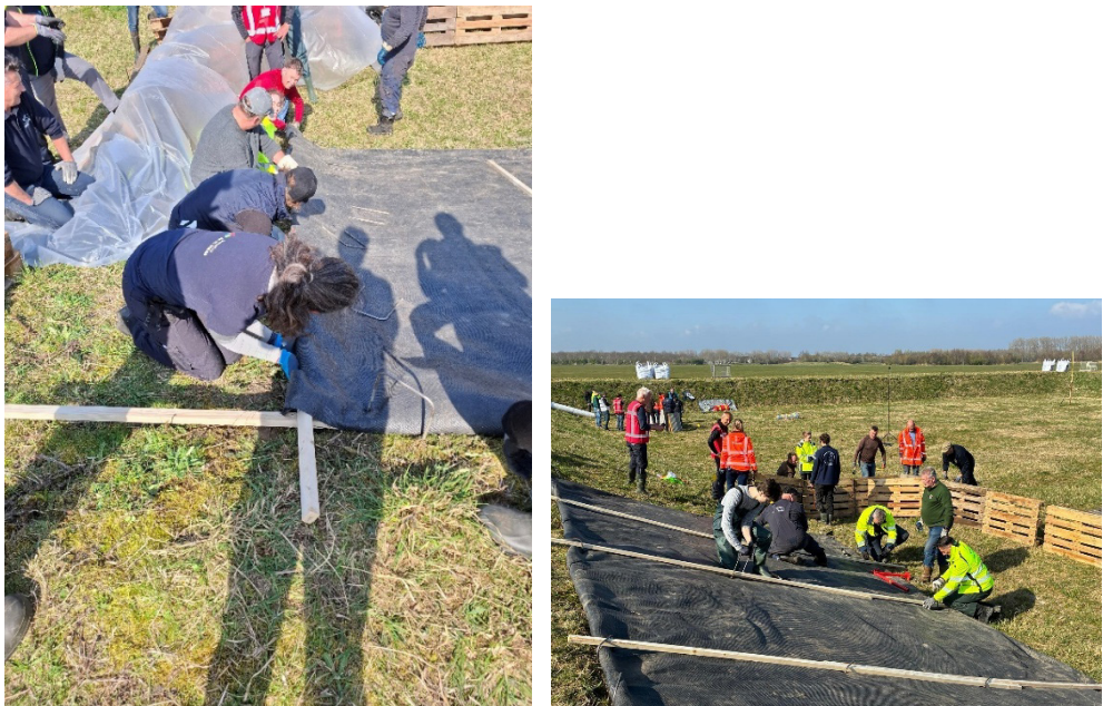
Figure 3.11 Left: timber batten being rolled into the side edge of the fabric. Right: timber battens positioned on the fabric and anchored to the ground using U-shaped staples.
