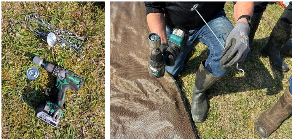
Figure 3.7 Gripple ground anchors installed using a specialised adapter for a cordless screwdriver.
