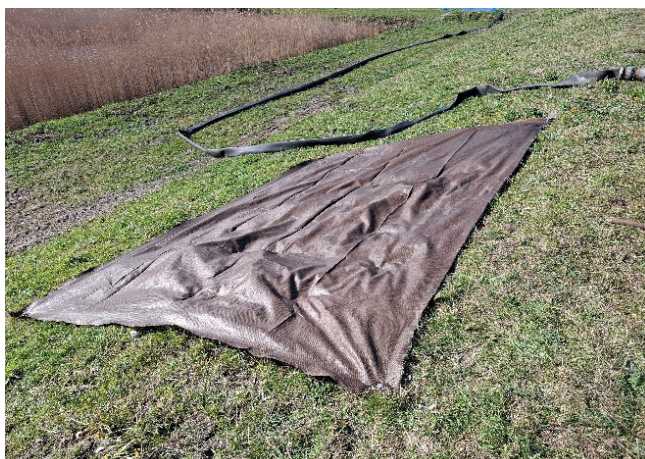
Figure 3.2 Biodegradable erosion-control fabric fixed to the ground at the corners using screws. In operational applications, wooden pegs are typically used instead.
