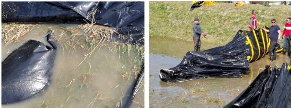
Figure 2.46 Residual water remaining in the TubeBarrier after drainage. The remaining water significantly increases the weight of the system, making handling and repositioning difficult.
