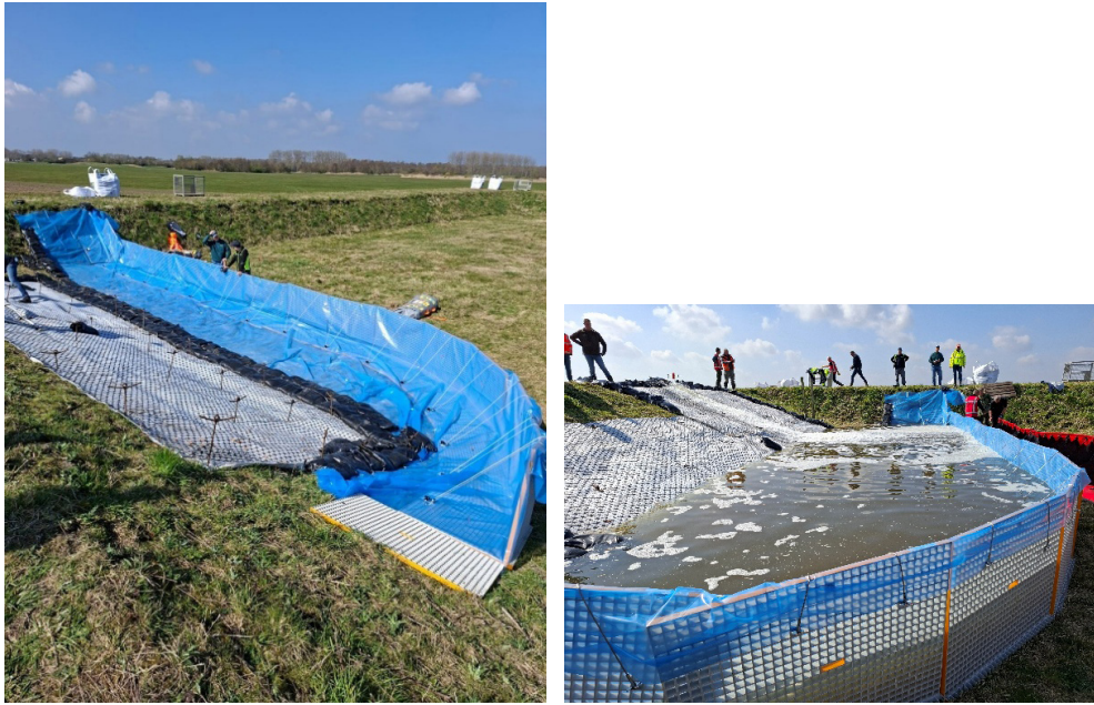
Figure 2.59 Water filling of the curved Haawal barrier configuration.
