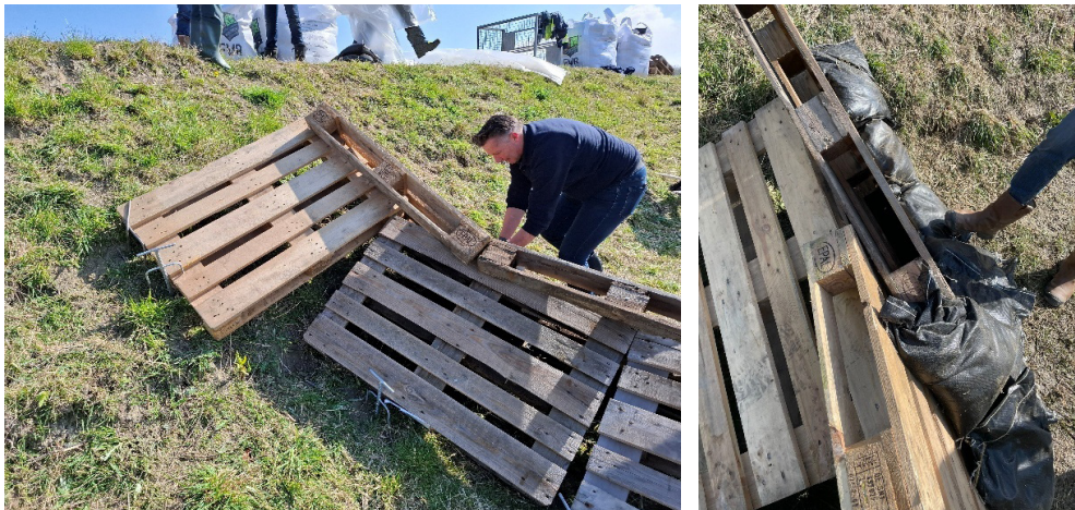
Figure 2.22 Placement of the Euro pallets at the slope transition is more challenging because the elements do not interlock properly in a staggered bond arrangement. Sandbags are required to seal the gaps to the ground surface and provide stability, while the pallets are secured together using steel staples.
