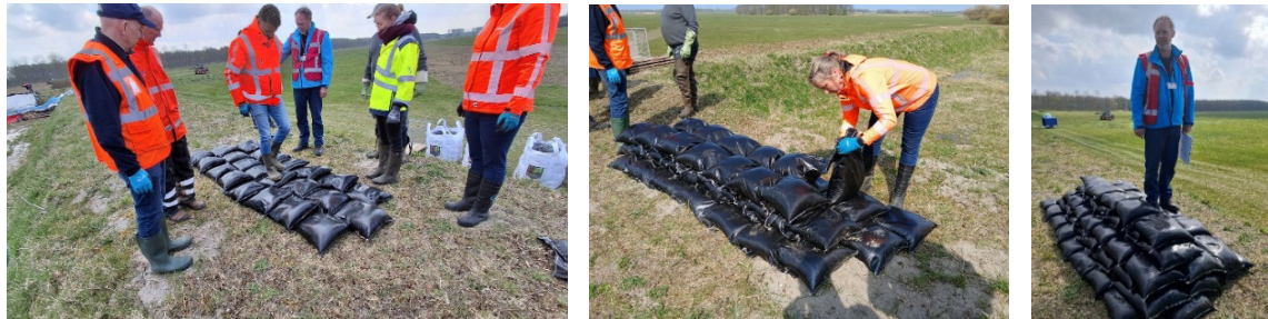
Figure 4.3 The first layer of sandbags is installed with the tail of each bag overlapping the head of the preceding bag. Successive layers are placed in a staggered bond pattern, with the second and third layers offset relative to the first layer and the fourth layer offset relative to the third layer.
