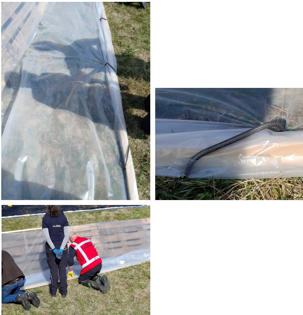
Figure 2.25 The opposite end of the plastic sheeting is rolled around timber battens and fixed to the ground using steel staples. The sheeting should be laid flat on the ground surface, avoiding trapped air and wrinkles as much as possible.
