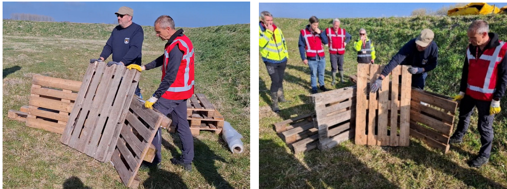
Figure 2.13 To enable curved sections or 90-degree changes in direction, an additional pallet is placed on its narrow edge at the corner location. The spaces between the pallets are filled with sandbags to ensure stability and continuity of the structure. The impermeable sheet should additionally be clamped beneath the pallets to prevent uplift of the sheet under hydraulic loading.
