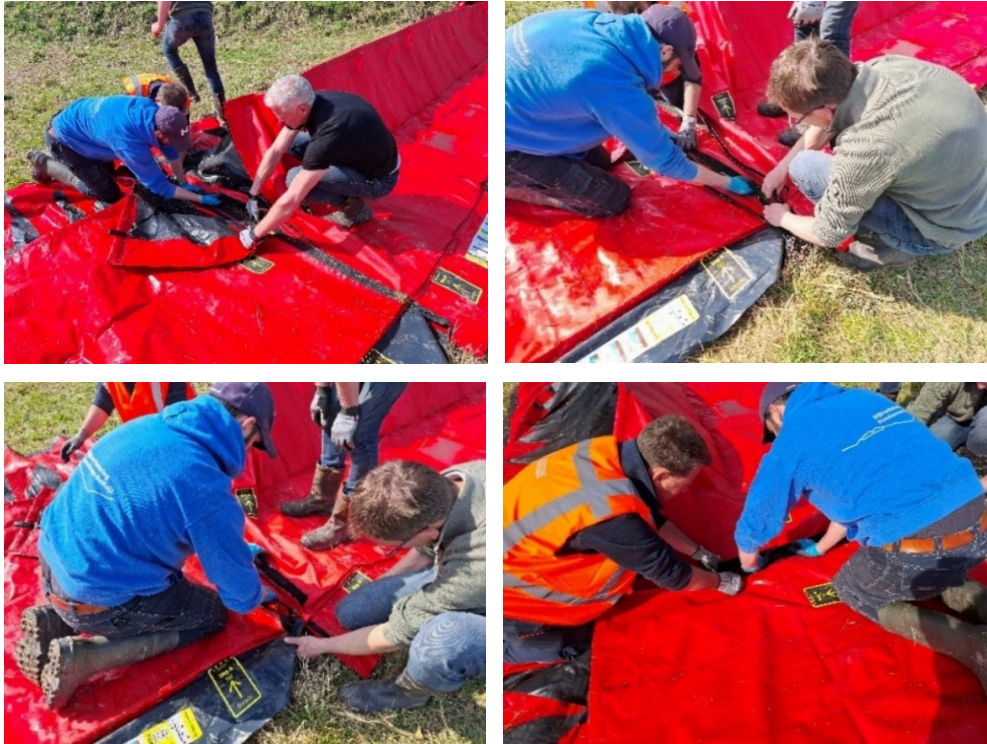
Figure 2.76 To maintain the BFW system in its deployed configuration prior to filling, support brackets are installed to keep the structure upright in the absence of water.
