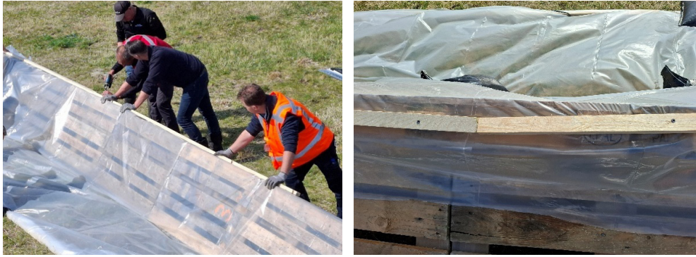
Figure 2.24 The plastic sheeting is secured at the top of the two-pallet system using screwed timber battens.
