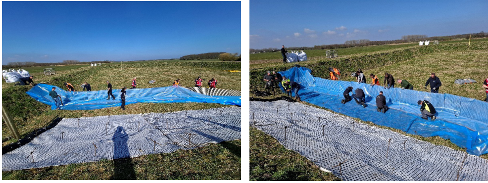
Figure 2.56 Placement and unfolding of the waterproof membrane and pressing it into the internal corner.
