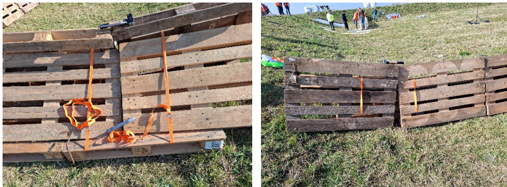
Figure 2.14 Each three-pallet module is held together by ratchet straps wrapped around the entire module. Left: supported side; right: the same situation viewed from the water-retaining side.
