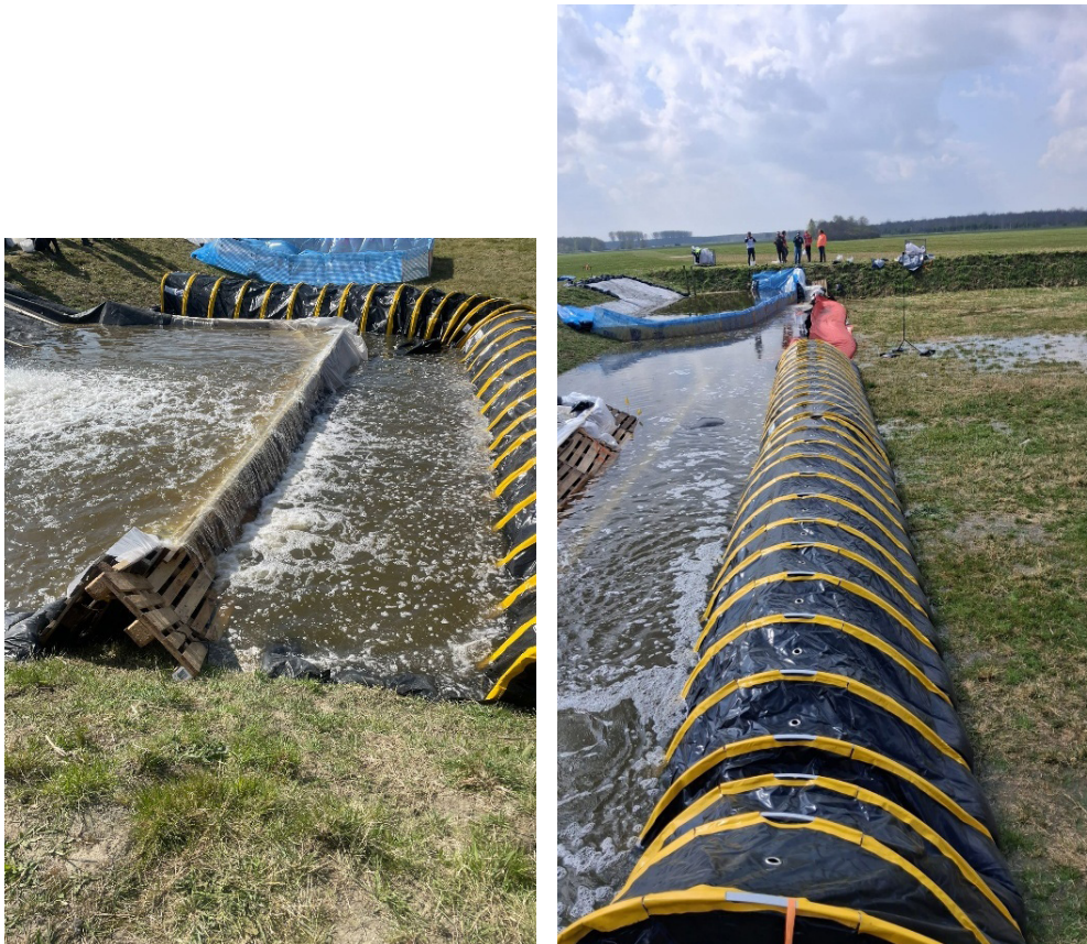
Figure 2.44 The space between the Euro pallet barrier and the TubeBarrier was filled with water. The ground surface on the protected side of the TubeBarrier showed clear signs of saturation due to underseepage beneath the barrier.
