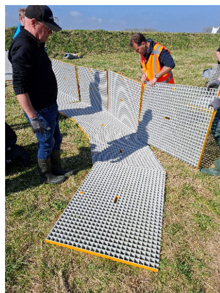
Figure 2.52 Installation of the Haawal system with a curved alignment.
