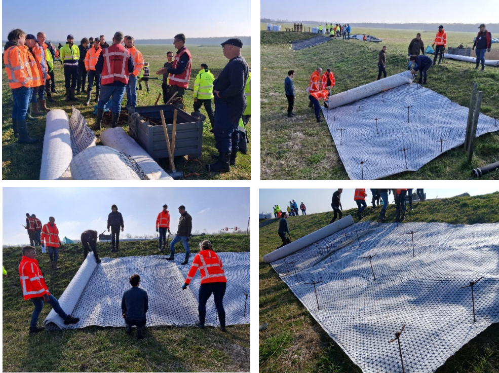
Figure 3.16 Tensar geogrid reinforcement secured with Y-pins. The overlap between two geotextile sheets is fixed using U-shaped staples, while sandbags are used to press the sheet edges against the ground.
