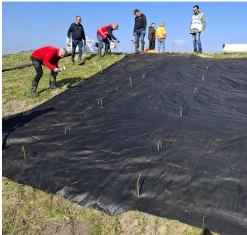
Figure 3.19 The geotextile is anchored by means of a high-strength rope that is looped around the anchoring pins. The rope is secured to an initial pin and subsequently unwound from the spool while being stretched across the geotextile surface.
