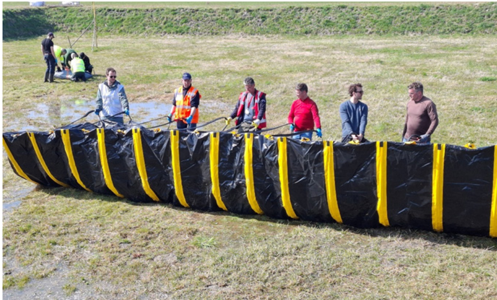
Figure 2.45 After completion of the test, the TubeBarrier system was disassembled. The process required substantial manpower, as the tube first had to be fully drained before the system could be removed and packed.
