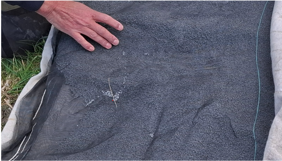
Figure 4.12 Sand Boil Filter Kit, including a schematic illustration of its operating principle.
