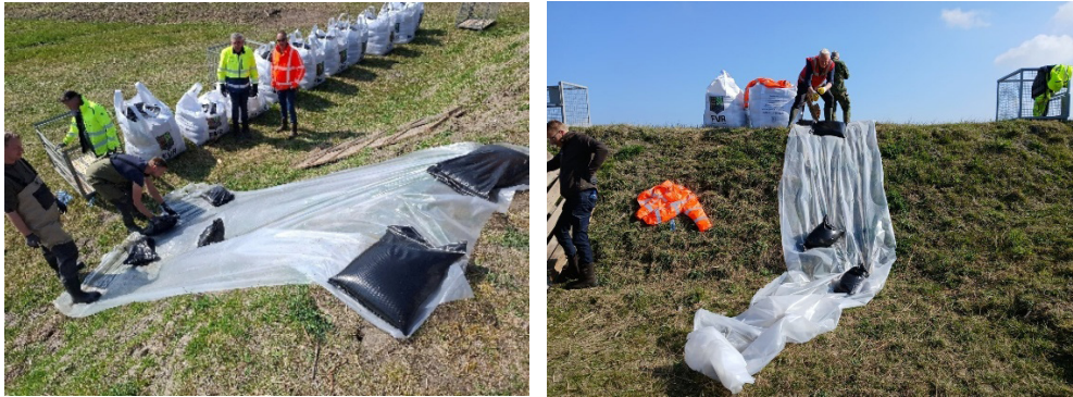
Figure 4.2 A membrane, ballasted at the crest with sandbags, is used as a chute to facilitate the transport of sandbags to the toe of the dike slope.
